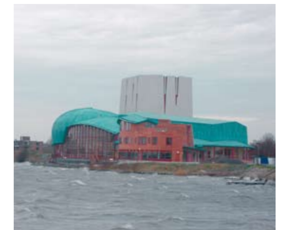
Theatre (The Netherlands) A very interesting example of the alkorPLAN® "copper" colour. Please note that only the main hall has been waterproofed with alkorPLAN® membranes, the rest of the building is covered with real copper.
