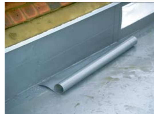
fig. 3: Edge restraint with alkorPLUS® 81170 or 81171 metalsheet
