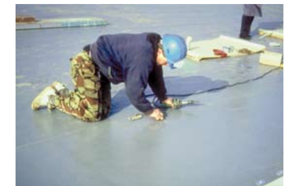
fig. 2: Verification of weld security
